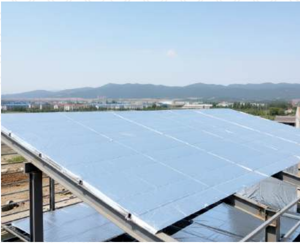
Step 1 : Unroll from ridge to eave, stretch firmly, and fix using drilling screws.
