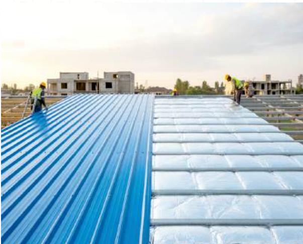
Step 3 : Match the next sheet, overlap cleanly, staple firmly.
